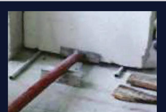
6. Use lever to lift ZMARTBUILD WALL PANEL until top of the panel reachthe upper floor then insert a wood wedge under the panel.
