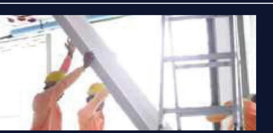
8. Apply thin-bed mortar on side of the first panel then lift the next wall panel to attach and do the same as the previous steps.
