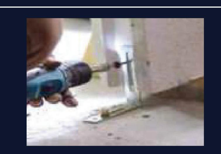
10. Measure the gap and cut the last panel to fit in then install it in place.
