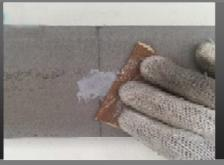
To conceal screw head, use wood filler, Leave to dry and rub it with sandpaper until the surface is smooth and even with the trim surface.
