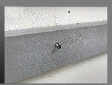
Insert needle point screw no. 10 (3 inches long) to plastic insert no. 7 before securing it into the hole. Hammer the plastic insert into the wall leaving the head in 1-2 cm.
