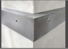
2. 45 degree angle cutting Install and conceal joint with wood filler and SCG Wood Substitute Acrylic Paint Sealant.
