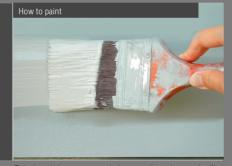
Painting: It is recommended to use the primer paint first and paint with SCG Acrylic Paint for Fiber Cement twice. Remark: Using oil paint with fiber cement material is not recommended.
