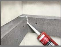
Finish up the work, especially in the corner and joint between the trim and wall with SCG Wood Substitute Acrylic Paint Sealant.
