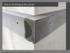
1. 90 degree angle cutting Mix concrete to fill the trim using brick trowel. Then, finish up the work.
