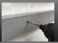
Use chalk line reel to indicate line. Then, place SCG Trim to the wall and use rotary drill with drill bits size 6.5 mm to make a hole on the concrete wall following the hole on the trim. Try to avoid touching the trim.
