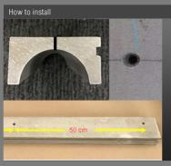
Make a hole on SCG trim with drill bits size 7 mm. To prevent breakage, do not use a hammering action. When hole is made, use drill bits size 10 mm to widen it 5 mm deep, to prepare for screw.
