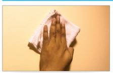
Clean surface before plastering, remove dust, stain or any dirt from wall. In case of plastering on mortar cement plaster, it should be repair some crack or hole before plastering
